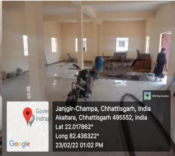
Library Reading Room (Under Construction)
